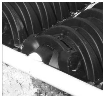
4. Secure lateral pipe to the top of the chamber.
