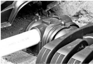
6. Insert connection pipe into endcap opening.
