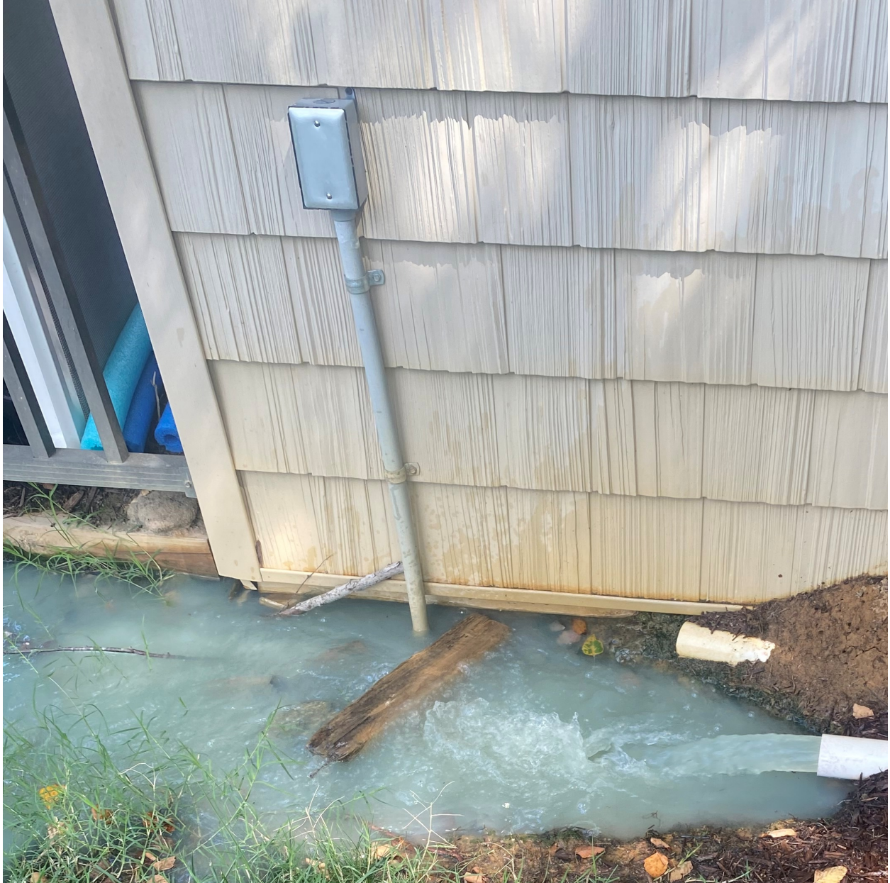
Figure 1. Backflush from apartment complex pool filter behind pool pump house
