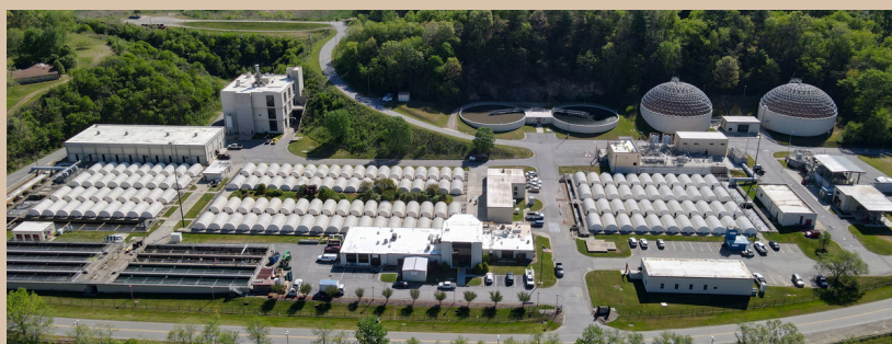
MSD Buncombe's Wastewater Treatment Plant
