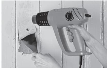
There is no way to eliminate dust, but some renovation methods make less dust than others. Contractors may choose to use various methods to minimize dust generation, including using water to mist areas before sanding or scraping; scoring paint before separating components; and prying and pulling apart components instead of breaking them.
